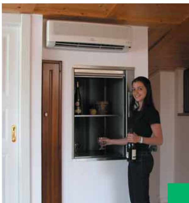
Installation in a private house (Italy), model 24 kg with stainless steel finishes. Thanks to Microlift the transport of goods from the garage to the kitchen is not a problem.
